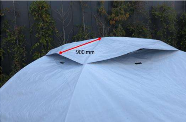
Picture 37: Top vents is located at 900mm from the roof centre
